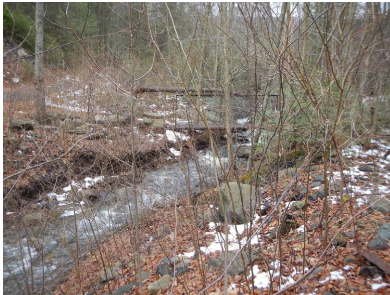
Pedestrian Bridge and Stream Bank Erosion along Reservoir Creek
