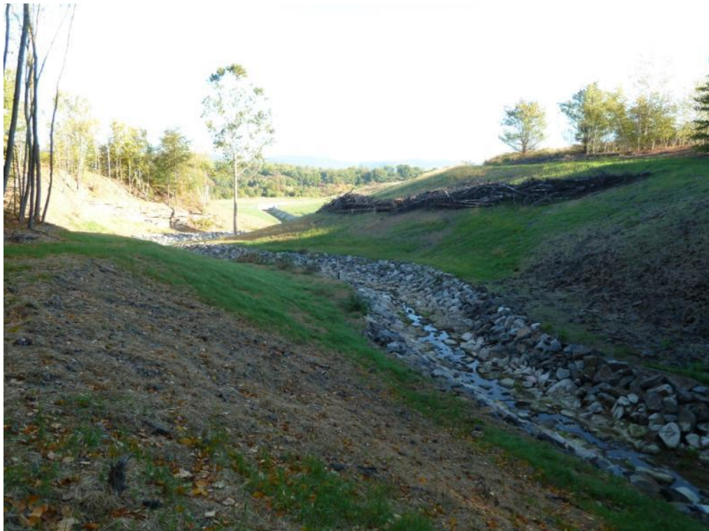
Grouted stream channel - Grading Area E looking towards Grading Area A
