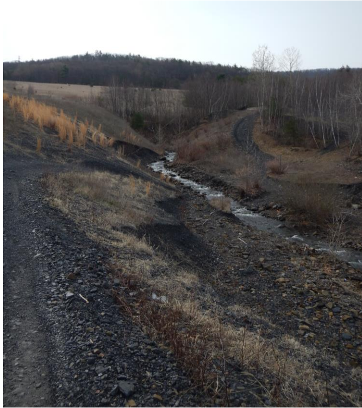
Stream Bank Erosion along Reservoir Creek
