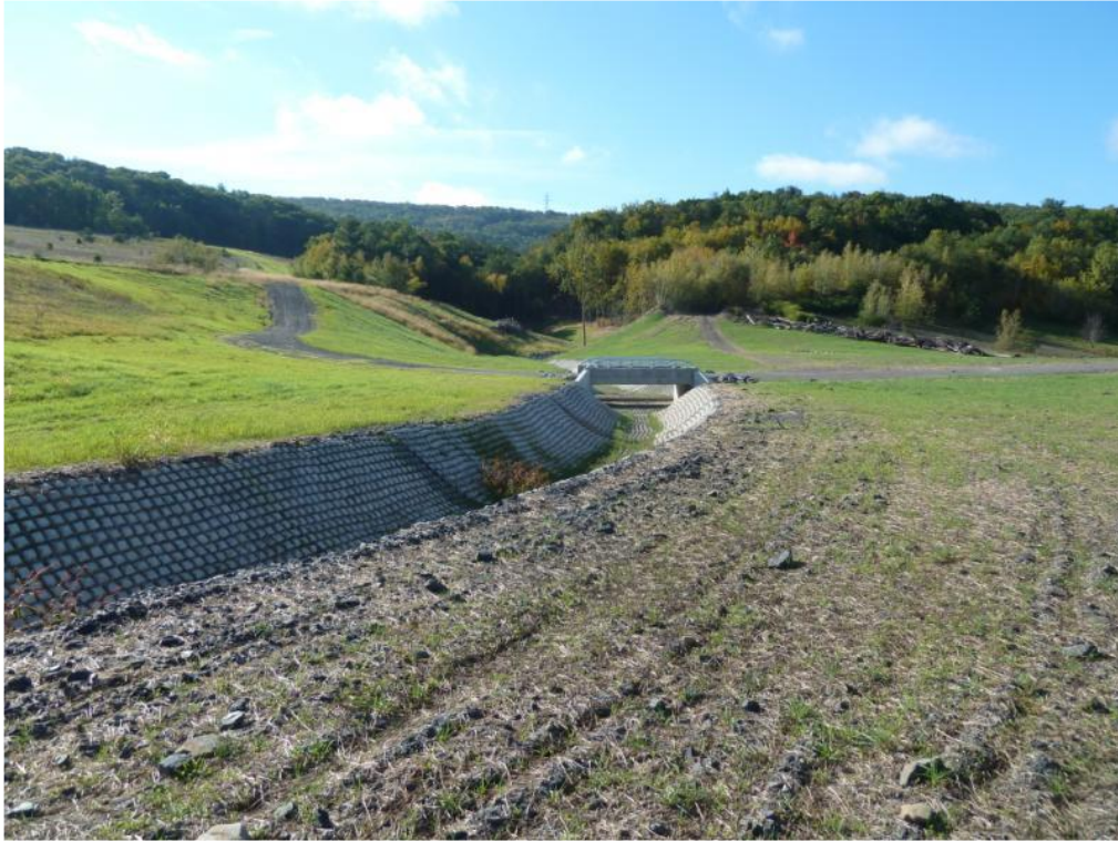
Box Culvert - Grading Area A looking towards Grading Area E
