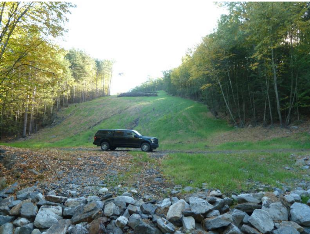
Site Disposal Area – Grading Area C
