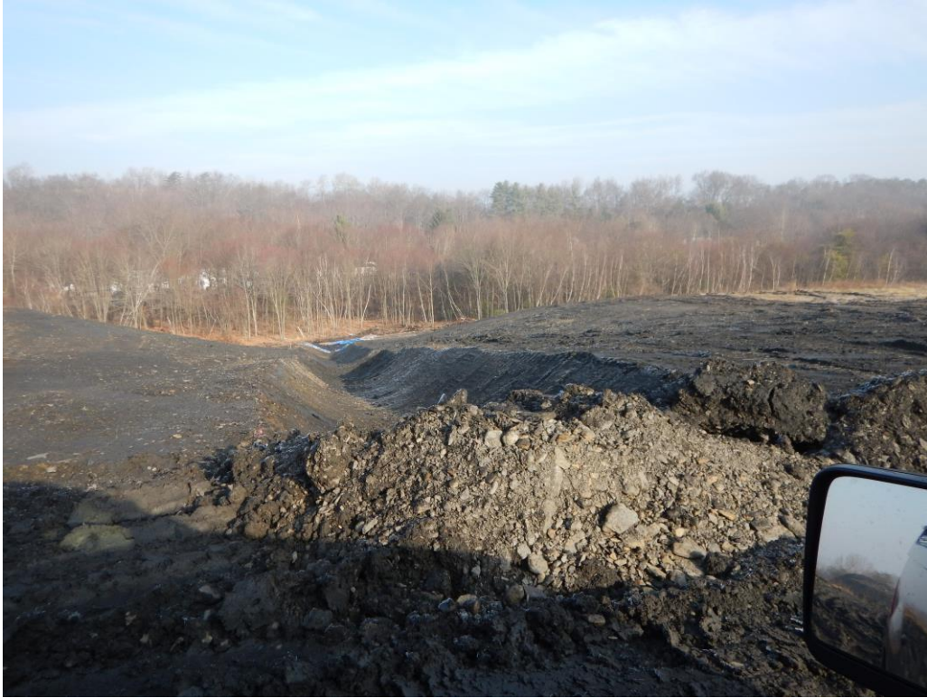
Channel Construction in Grading Area B
