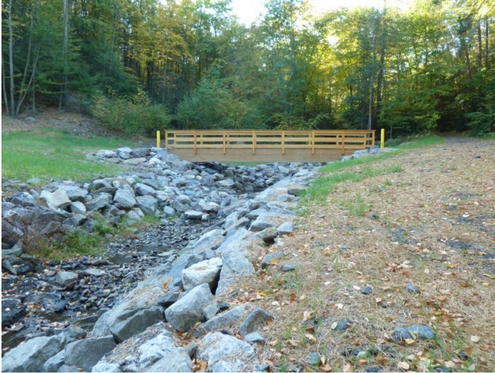
Grading Area C - Pedestrian Bridge - Grading Area D
