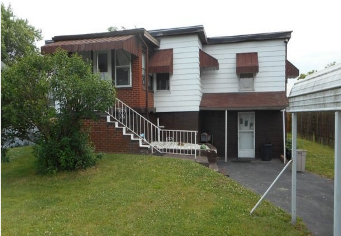
FAIRHOPE (MULTI-STRUCTURE SUBSIDENCE) CONTRACT NO. OSM 26(2757)102.1 EMER
