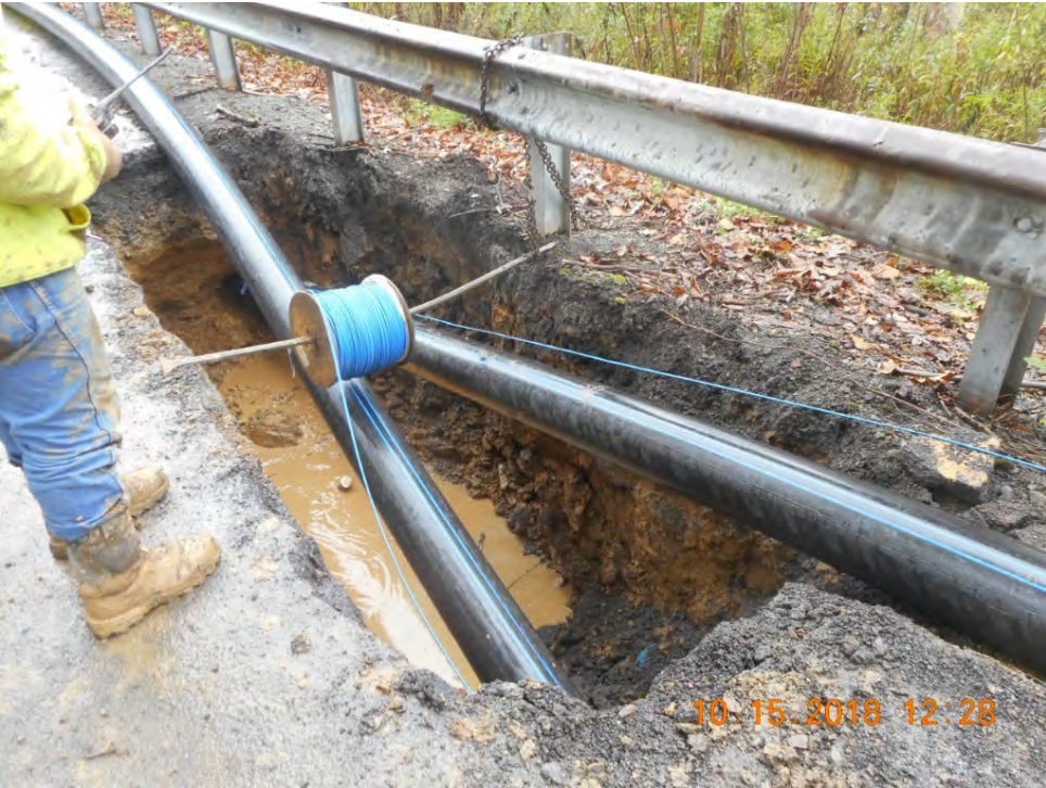
Installing waterline
