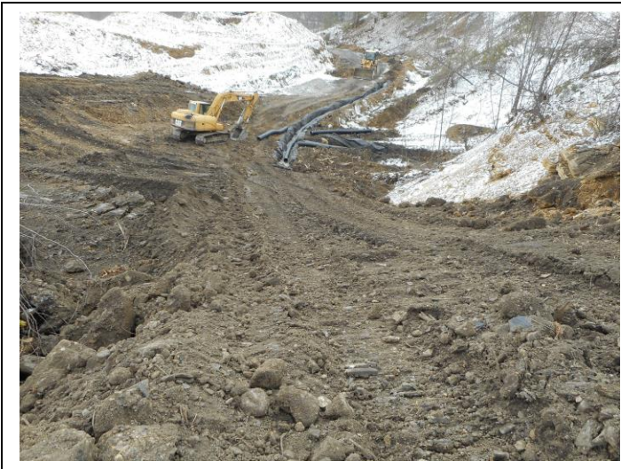
1/29/16 – Installing the 12-inch subsurface drain into the pit area on the southern end of the project site.
