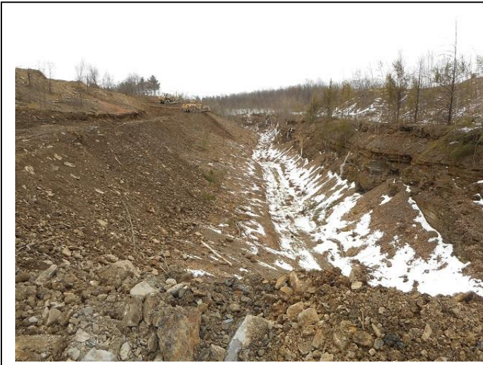
1/25/16 – Backfilling the pit and 60-foot highwall on the west side of the project site using two Cat D 11 dozers.
