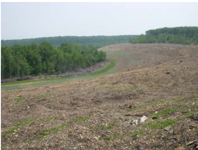
Final grade, vegetative filter strip and brush barrier at Area 2.
