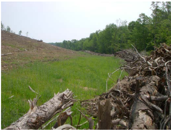
Vegetative filter strip and brush barrier at Grading Area 5.
