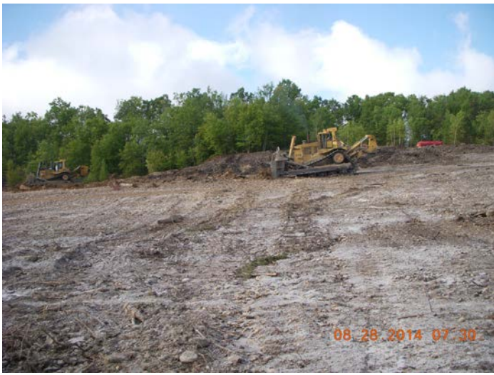
Incorporating lime at Area 4.
