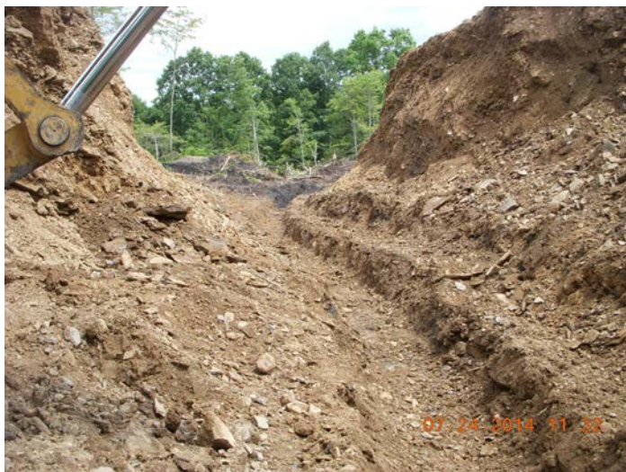
Underdrain excavation.
