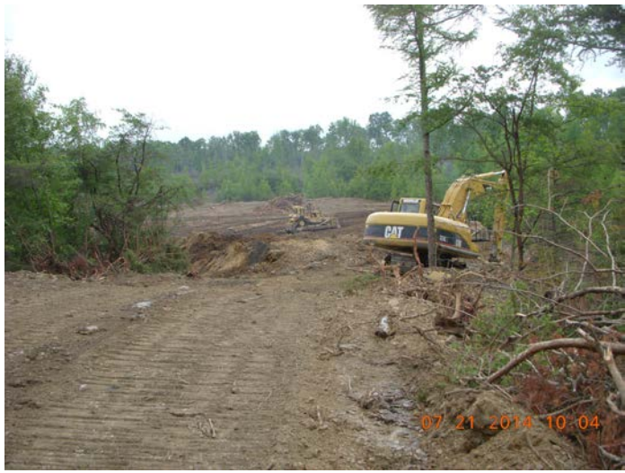
Grading at Area 2.
