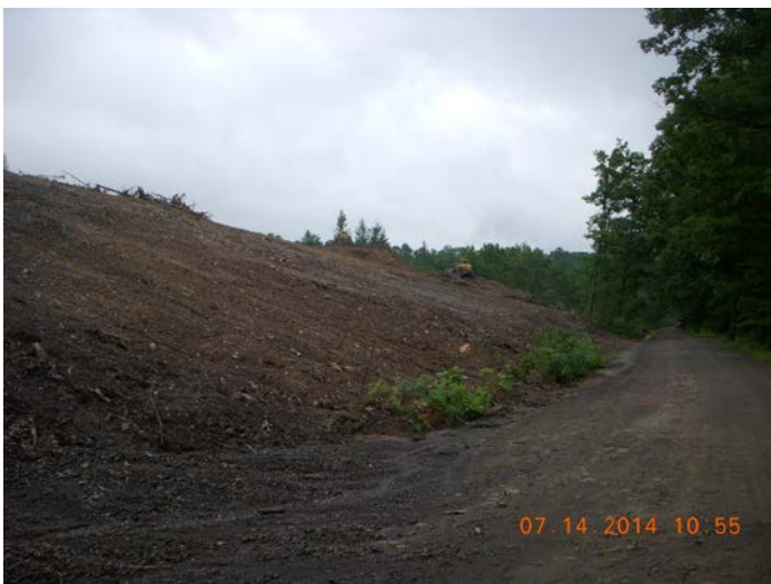
Grading at Area 2.
