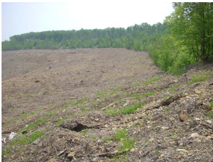
Final grade at Grading Areas 1 and 2.
