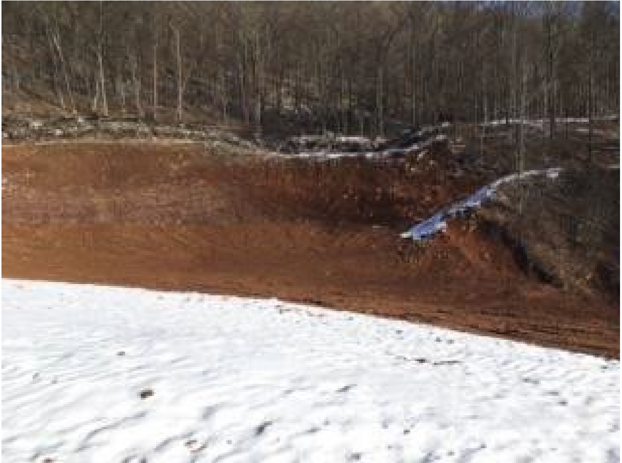
Subsidence Area Backfilled
