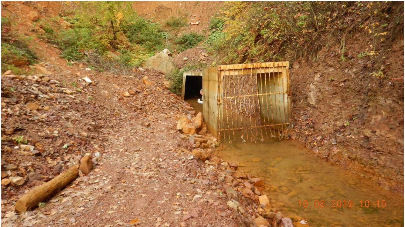
Downstream End of Existing Tunnel; Concrete Sections Separated
