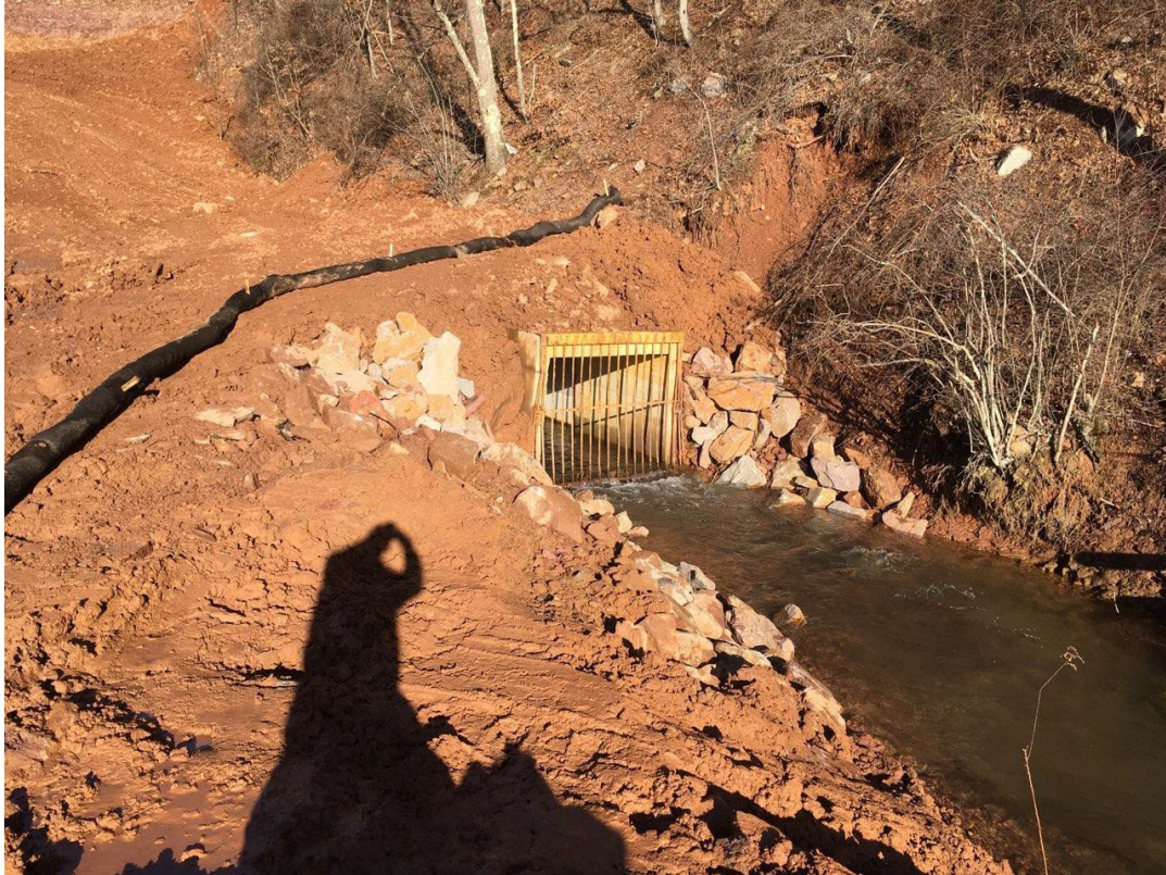
Extended Mouth of The Tunnel
