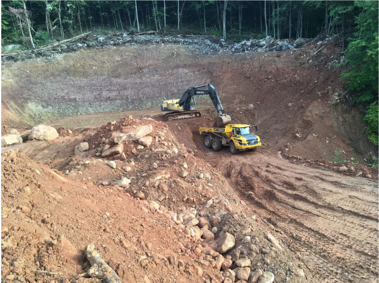
Excavating Subsidence Area
