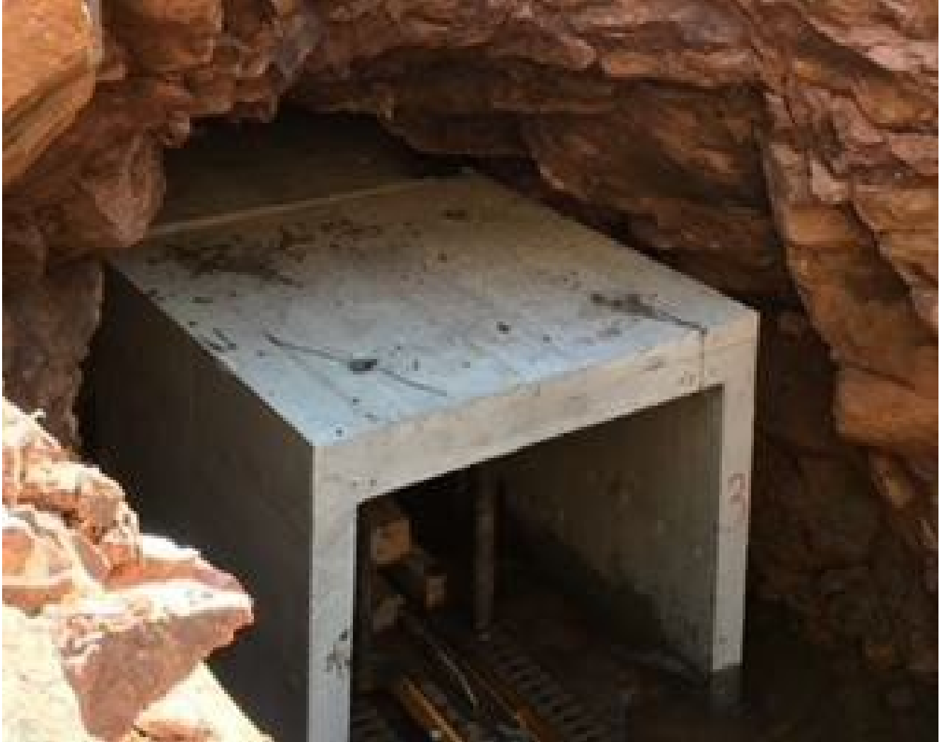
Placement of Concrete Sections Within Subsidence Area
