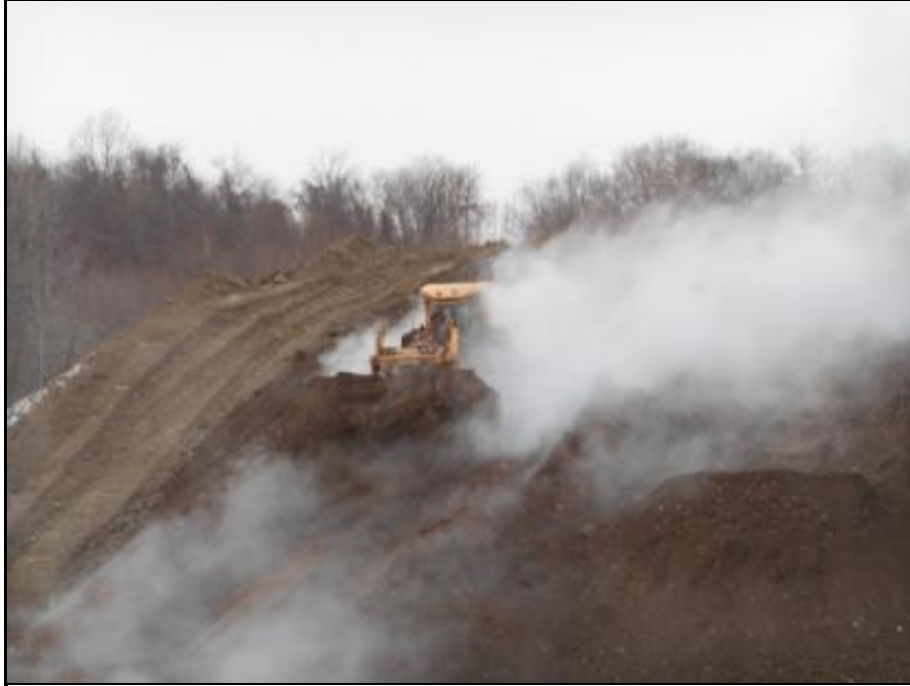
01/09/2015 - Excavation of project site
