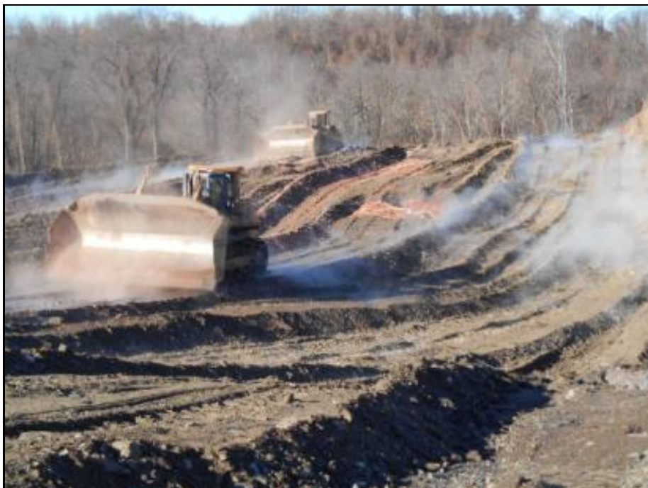
01/13/2015 - Excavation of project site
