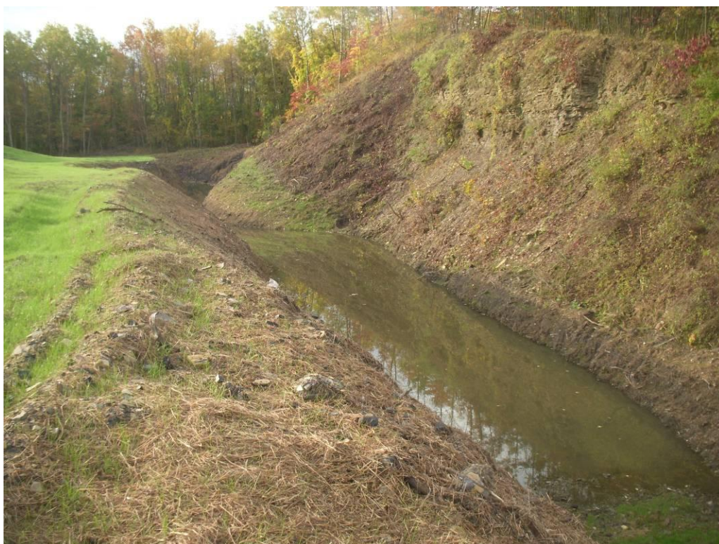
Completed isolation trench (2012-10-10)
