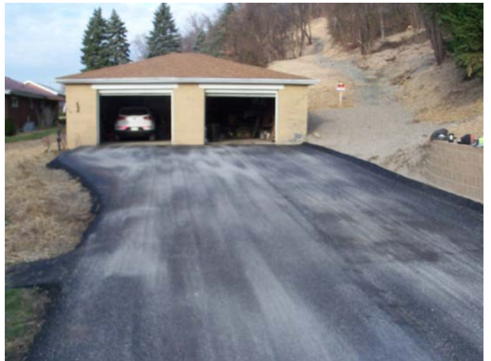
New driveway constructed by the property owner as a result of the project.
