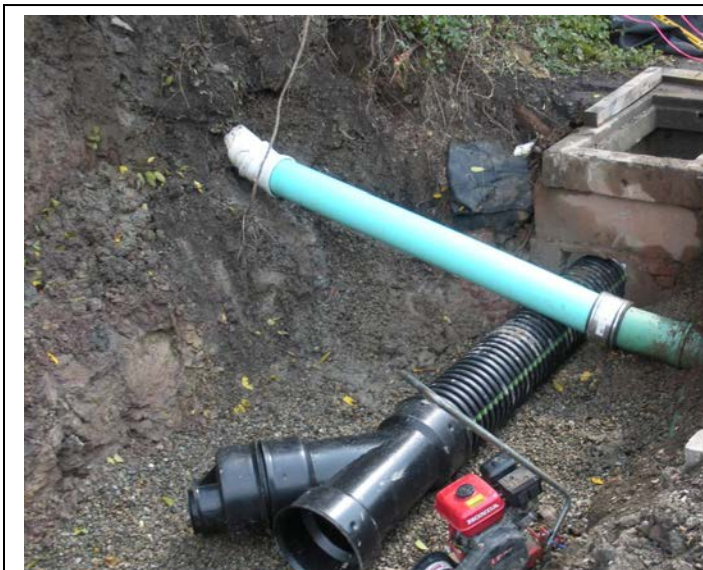
Connection into culvert at 2 nd Street.
