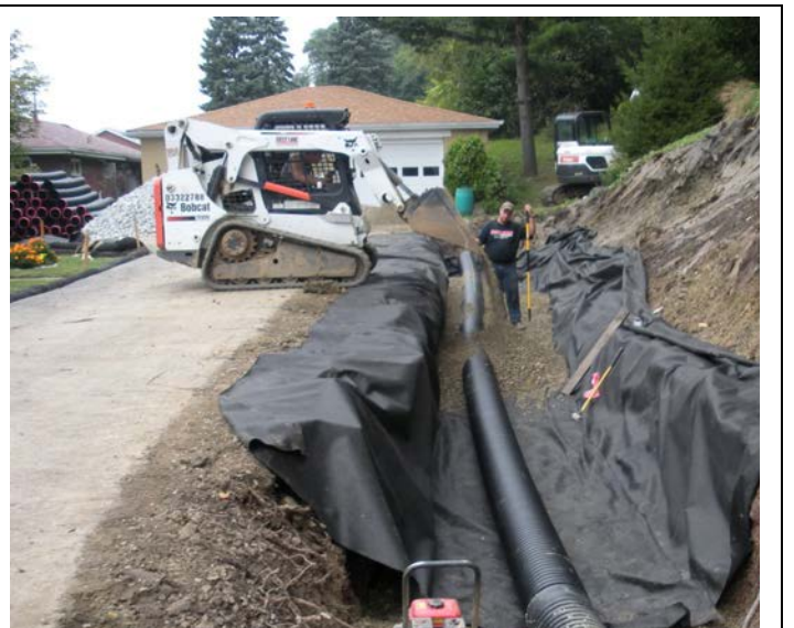
Main line along driveway at Ms. Semian's house.
