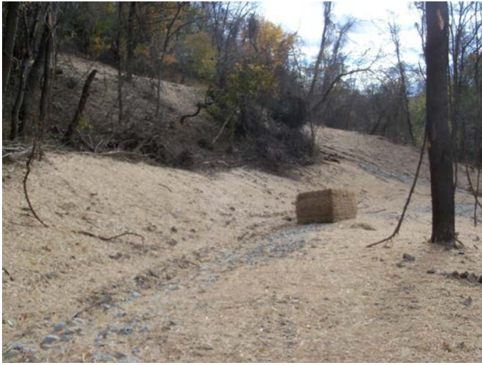
Seeding and mulching main drain line.
