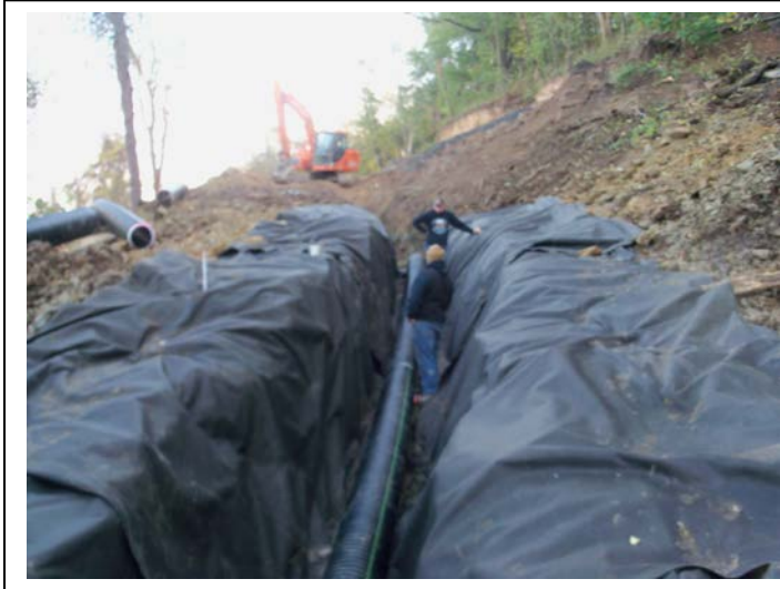
Typical look at laying pipe.
