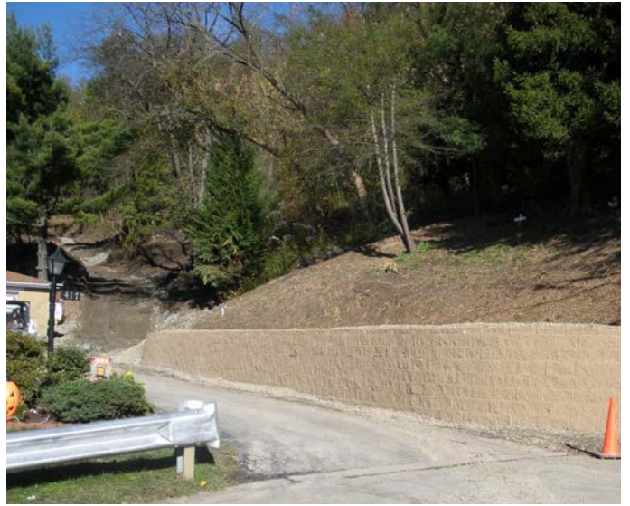
Wall constructed at Ms. Semian's home.
