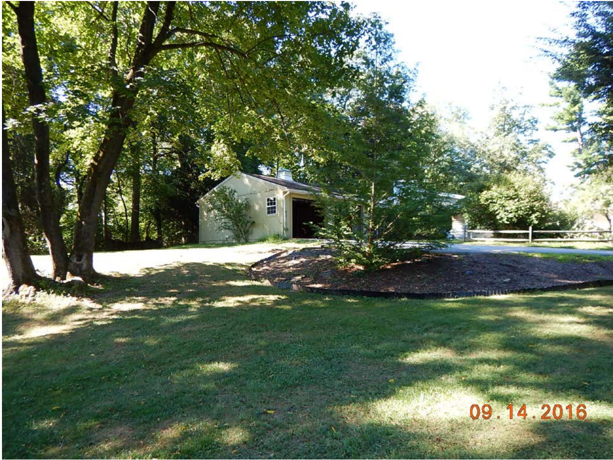
SUBSIDENCE OPENING SIDE OF ATTACHED GARAGE
