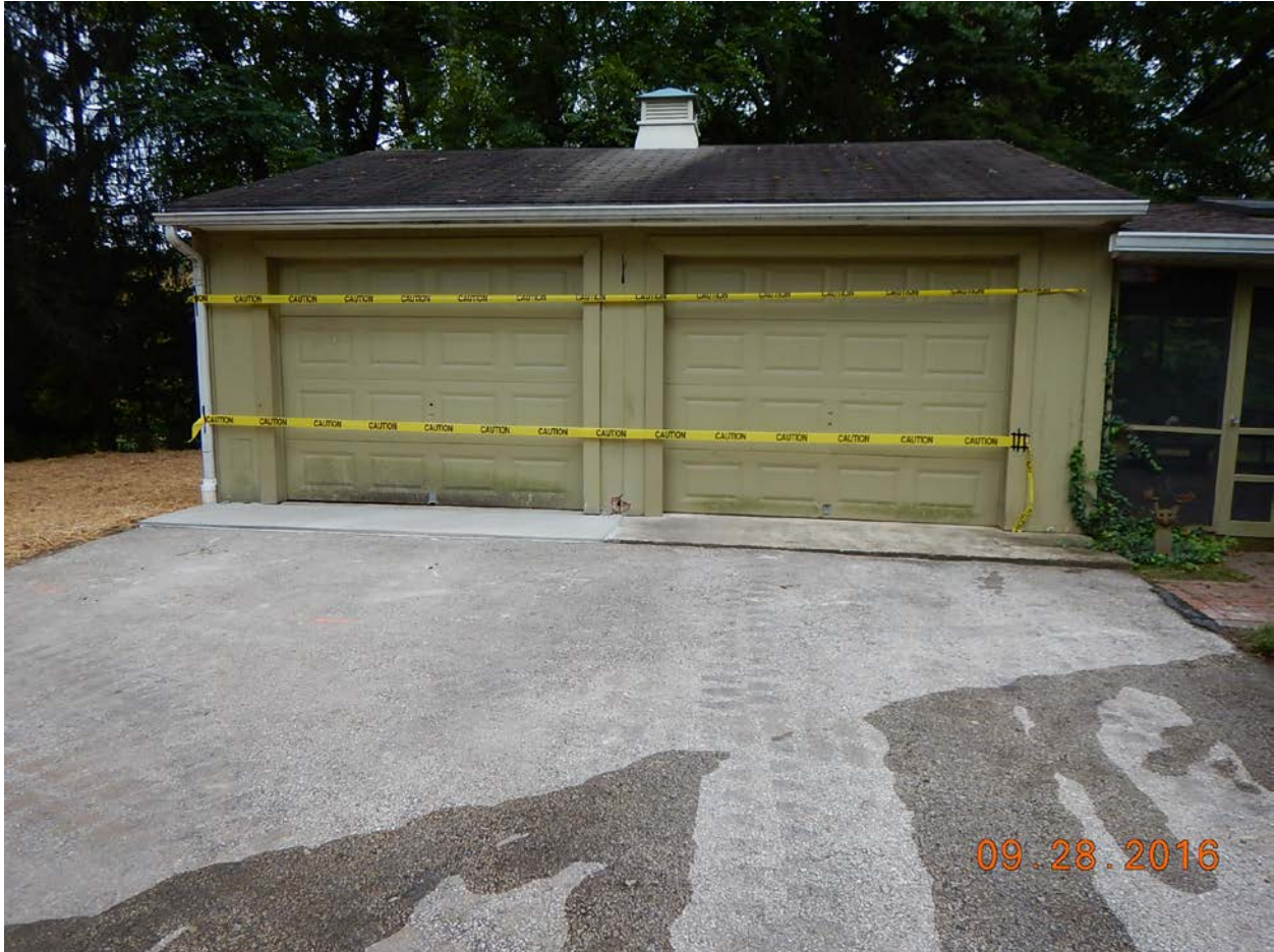
APRON REPLACED ON LEFT BAY OF ATTACHED GARAGE
