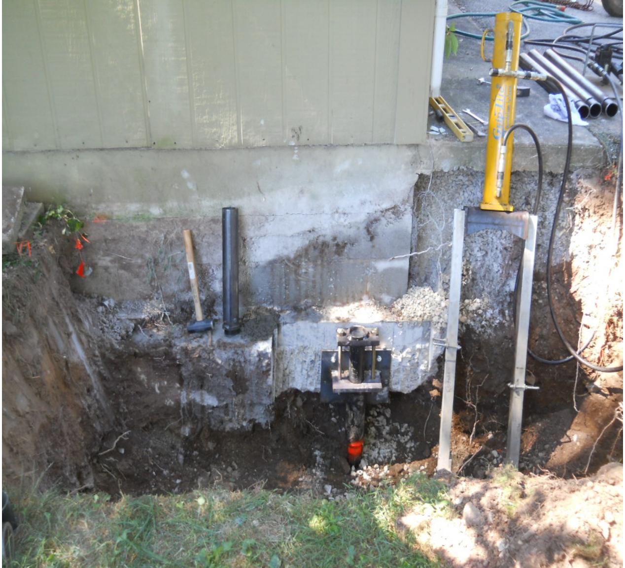
INSTALLATION OF STEEL PUSH PIERS TO SUPPORT GARAGE
