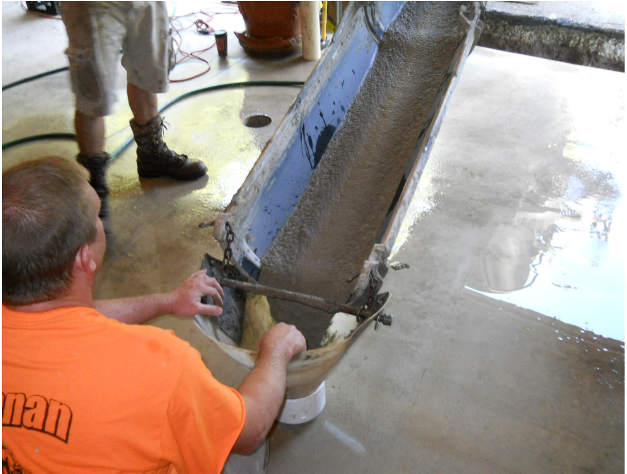
BACKFILLING MINE SHAFT THROUGH COREHOLES WITH FLOWABLE FILL
