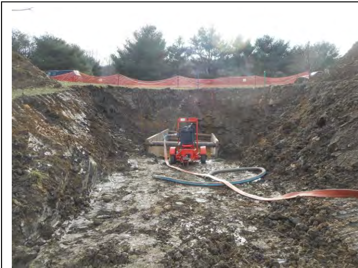
Excavating the mine seal
