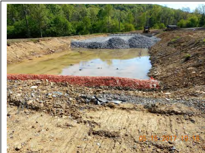
Constructing the horizontal limestone bed
