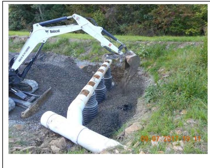
Placing limestone in the manganese removal bed
