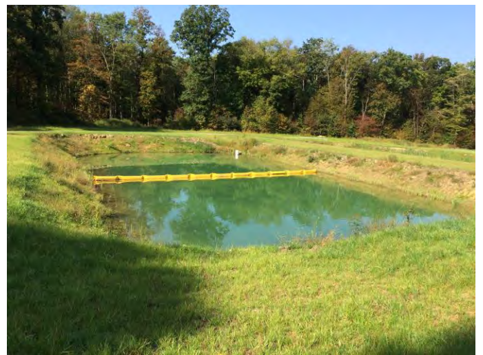
Settling Pond No. 2
