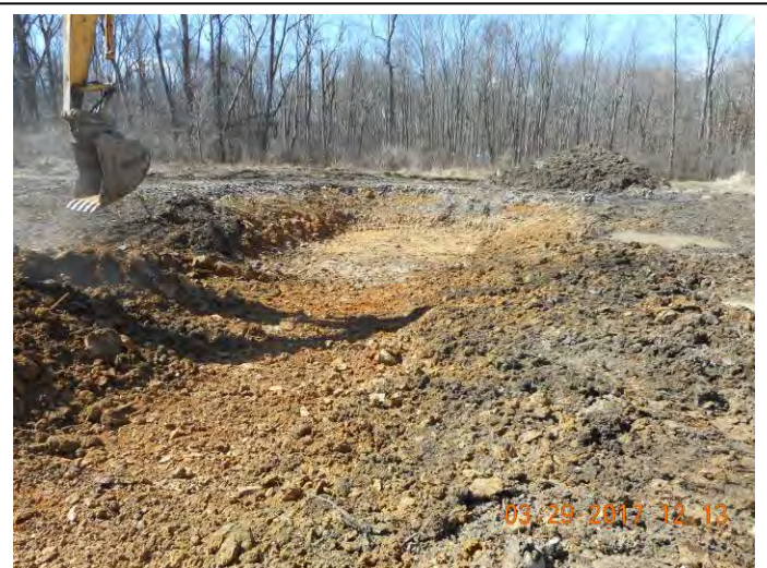
Excavating for Settling Pond No. 2
