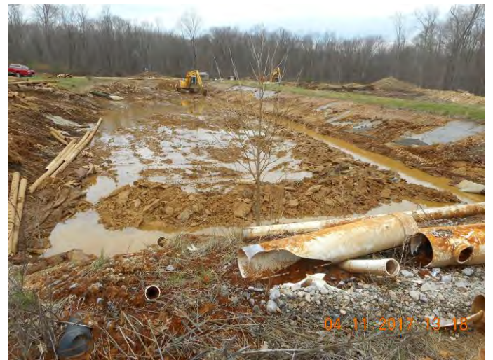
Excavating limestone and piping from the existing limestone upflow bed
