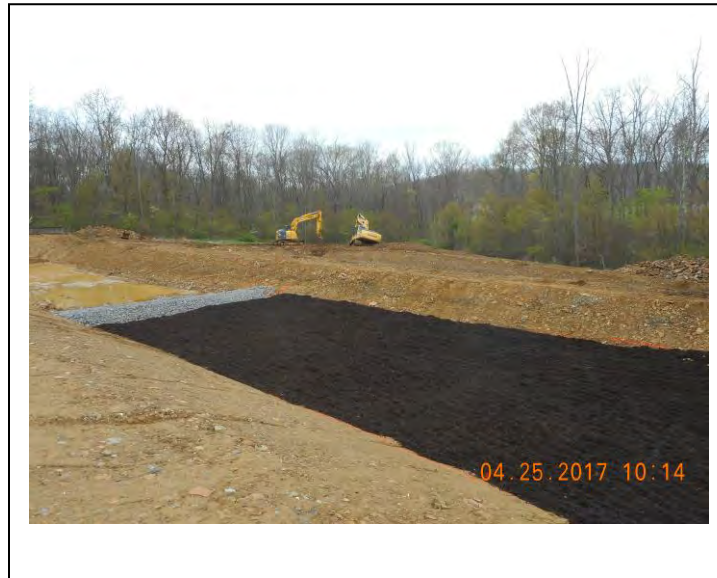
Constructing the aerobic wetland
