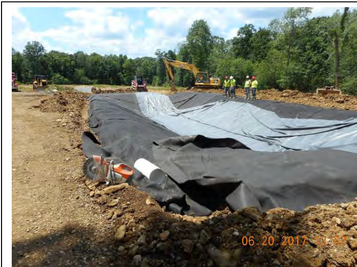
Constructing Settling Pond No. 1
