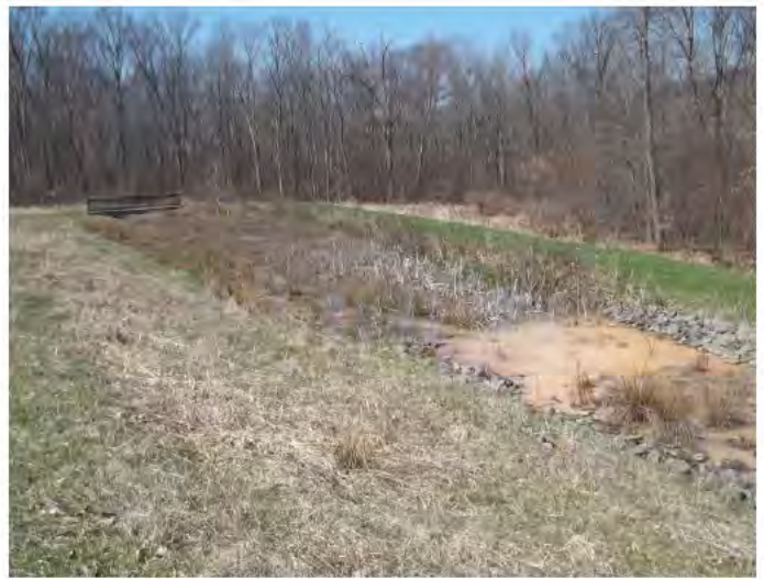
Flushing pond from the northeast embankment looking northwest
