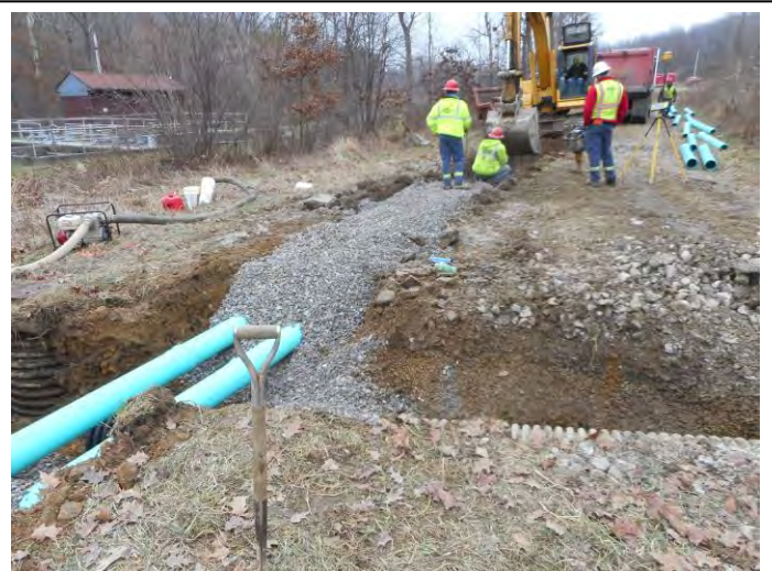
Placing new conveyance pipelines
