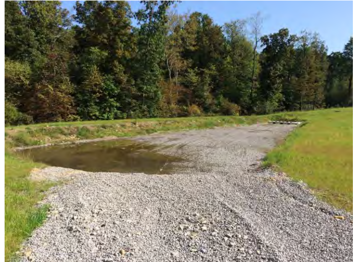
Manganese Removal Bed
