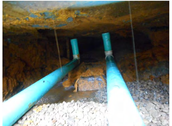
Installing dual mine drains
