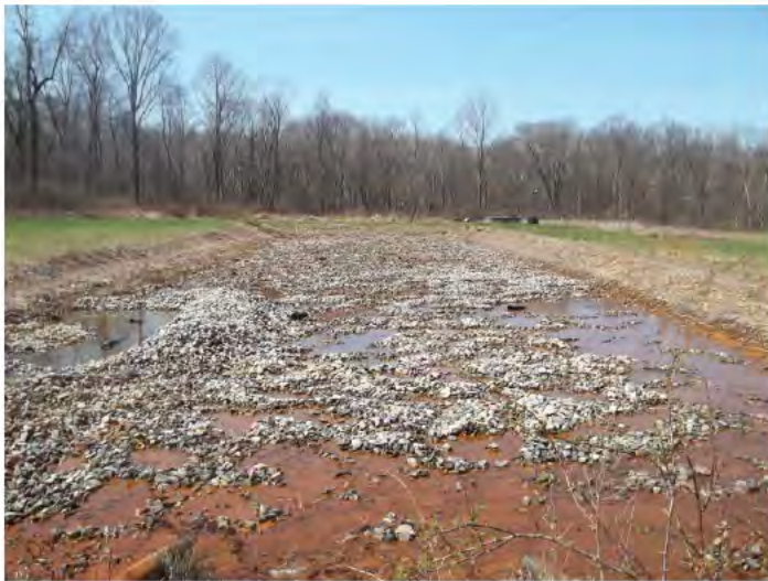
Limestone upflow pond from the center of the northeast embankment, looking southeast
