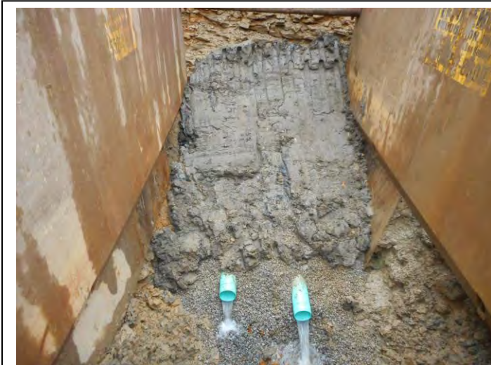
Clay mine seal and mine drains
