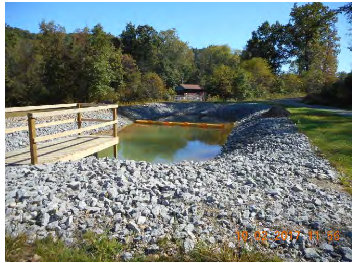
Settling Pond No. 1
