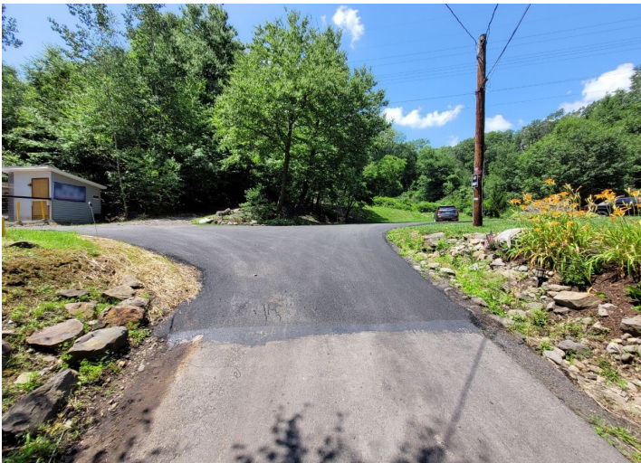
View of the joint between the new asphalt and the existing Sickler Hill Road
