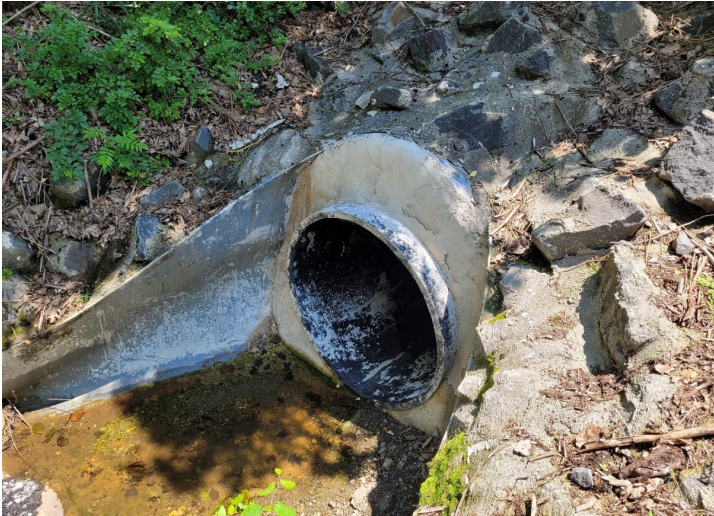
View of the upstream end of the installed pipe
