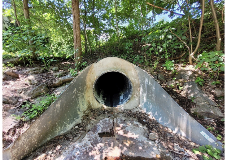
A view of the downstream end of the pipe after installation was completed
