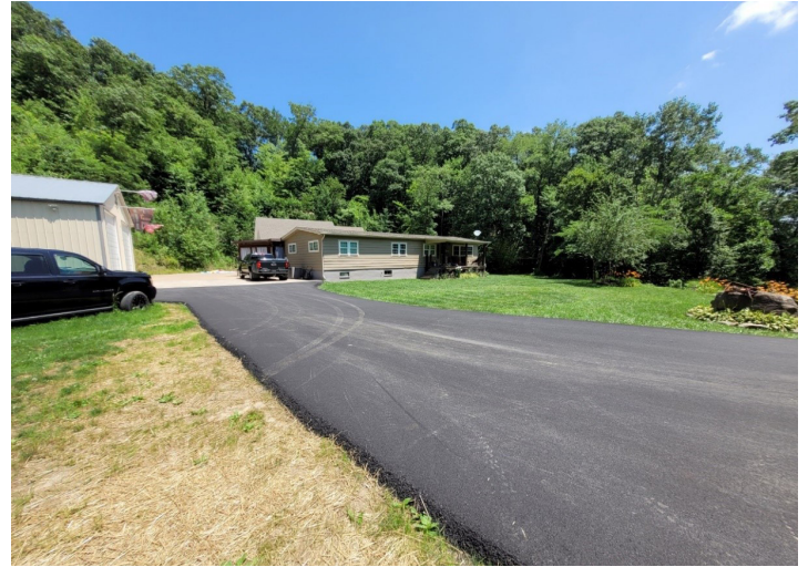
View of the new asphalt and residence at 130 Sickler Hill Road
