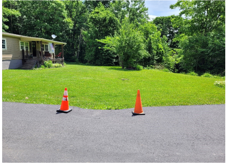
An alternate view of the subsidence in the driveway and the yard
