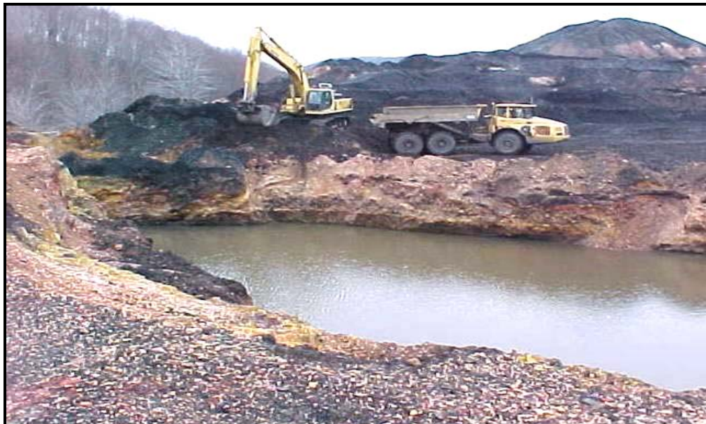
Barnes-Watkins project in construction: encountering river-level infiltration.
