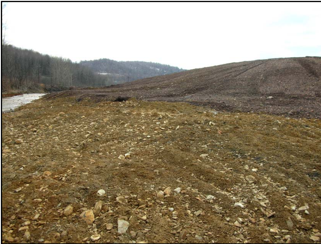
FBC ash being applied during reclamation.
