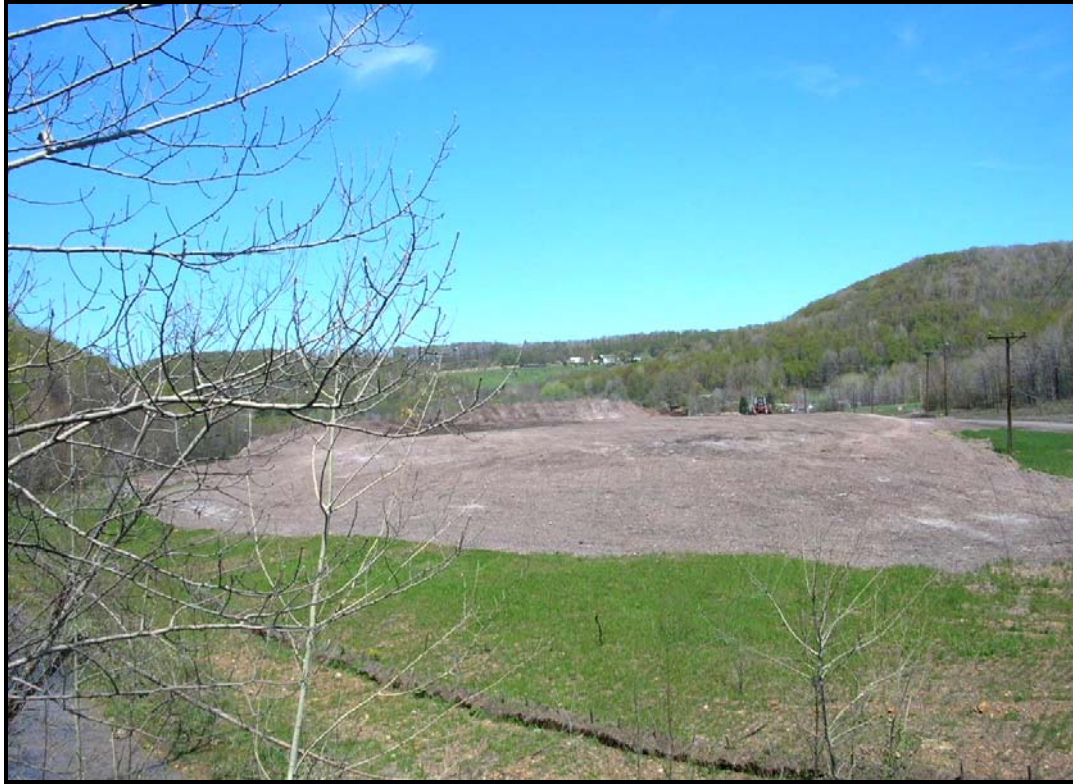
Completion of FBC ash application on Phase 1.
