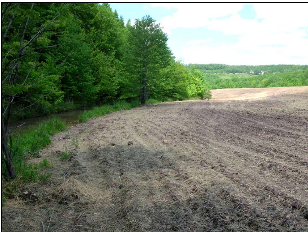
Completion of seeding at Barnes-Watkins site.
