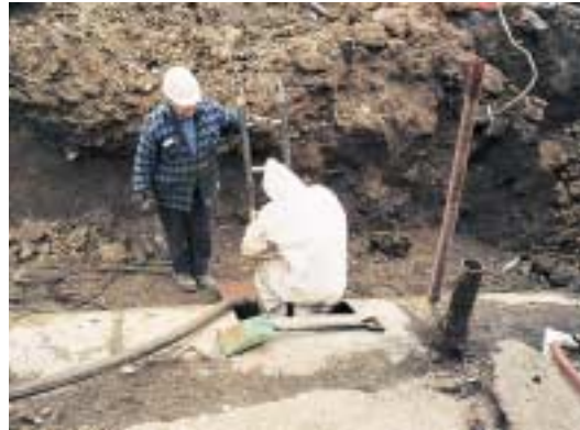
Petro Clean, Inc., inspector M. Hartley assesses an underground storage tank.
