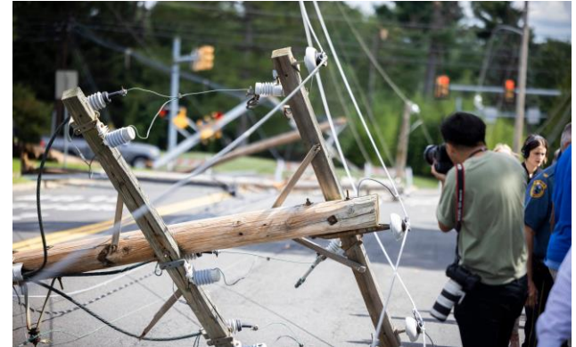
Damage from Hurricane Ida, Sept. 2021, southeastern PA
