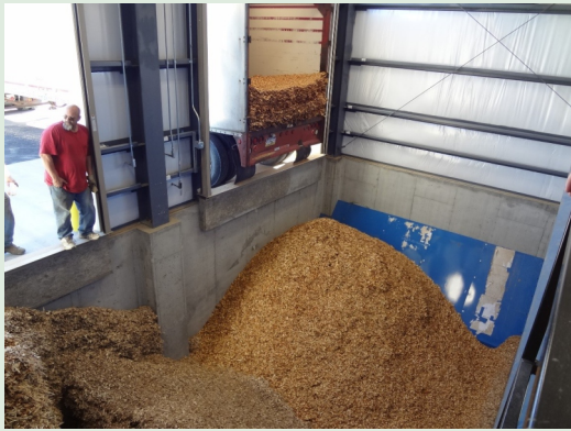
Wood chip storage, housed in a newly constructed building
