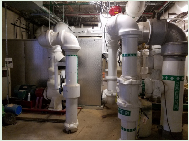
New chilled water lines
