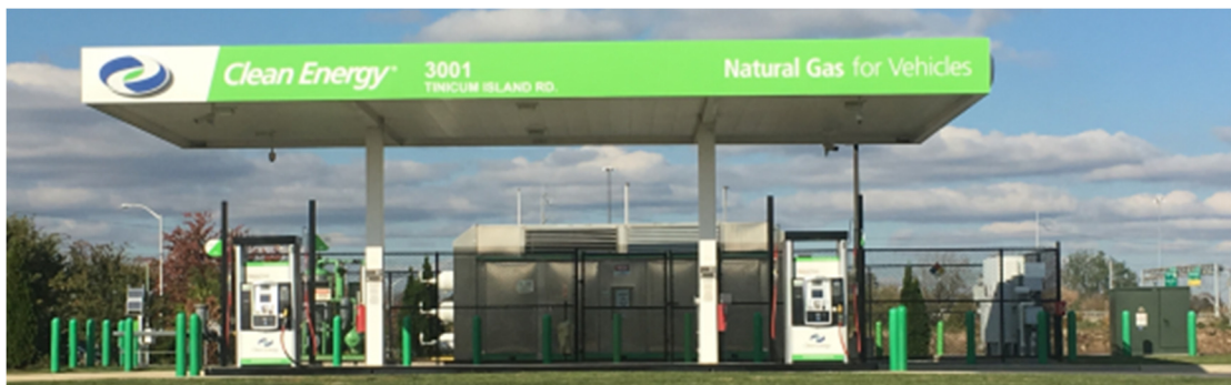
Figure 7 – CNG Fueling Station at Philadelphia Airport
