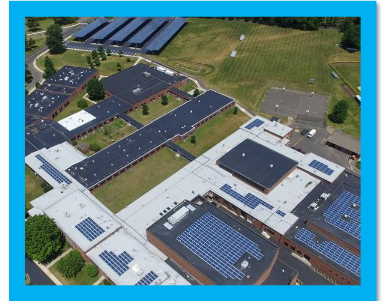
Energy & Frequency Regulation from Solar-Storage Microgrid
