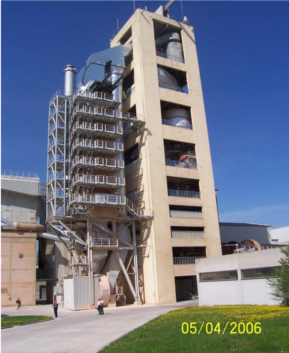
FIGURE 1 Solnhofen SCR Reactor sited next to preheater tower on right
