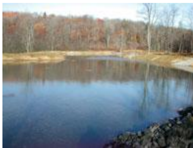
Figure 2-5. Another limestone treatment pond. Photo courtesy: Jon Smoyer, PADEP BAMR
