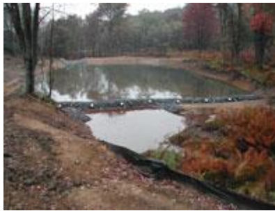
Figure 2-4. One of a series of limestone treatment ponds installed. Photo courtesy: Jon Smoyer, PADEP BAMR
