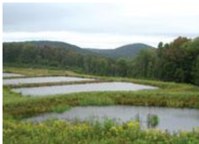
Figure 2-2. A portion of the Anna S. Passive Treatment System. Photo courtesy of PADEP
