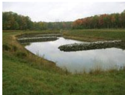
Figure 2-12. Settling pond with limestone baffles. Photo courtesy of Kay Spyker, PADEP BAMR
