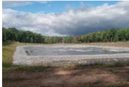
Figure 2-11. Vertical flow limestone treatment pond. Photo courtesy of Richard Macklem, Pennsylvania State Game Commission
