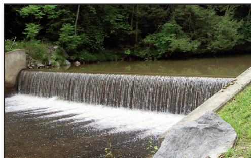
The dam on Larrys Creek. This dam was originally constructed from wood. The JSJWA replaced the wood with concrete in 1988.
