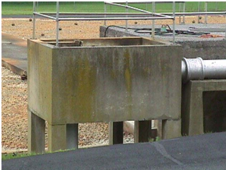
Figure 1.4 Dosing Chamber for Stationary Trickling Filters
