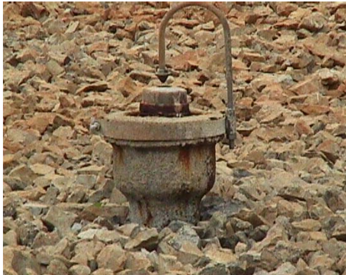
Figure 1.6 Spray Head for a Stationary Trickling Filter
