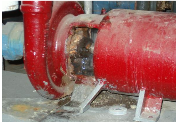
Figure 3.1 Leaking Gland
