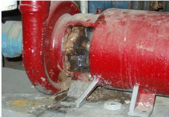
Figure 3.1 Leaking Gland
