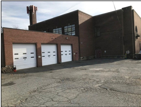
Borough's collection fleet storage facility
