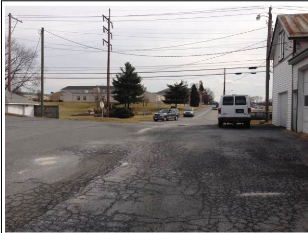
Photo 1: 02-15-13. Proposed Ewaste Building Access Road adjacent to building.
