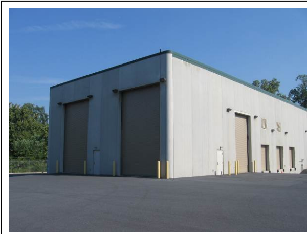
Photo 1: 02-22-13. Dauphin County Recycling Center. eWaste Recovery Program.
