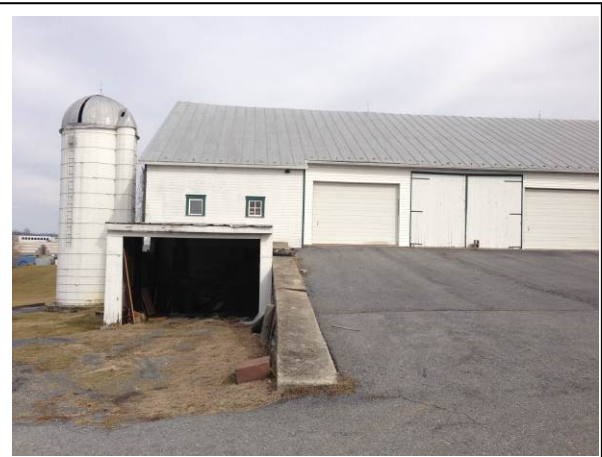
Photo 1: 02-22-13. Proposed Ewaste Building #2 Not suitable due to low ceilings and support beams.
