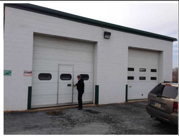
Photo 2: 02-15-13. Proposed Ewaste Building Overhead doors to building.
