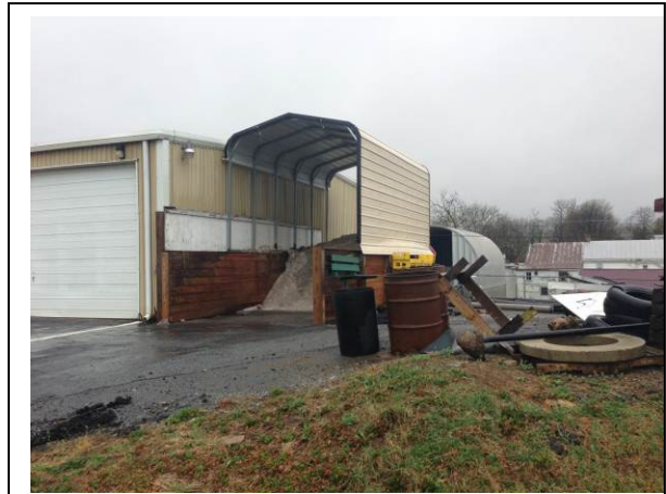
Photo 2: 02-22-13. 04-12-13. Newville Borough Salt shed across from electronics drop-off
