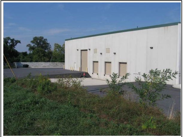
Photo 2: 02-22-13. Dauphin County Recycling Center. eWaste Recovery Program.
