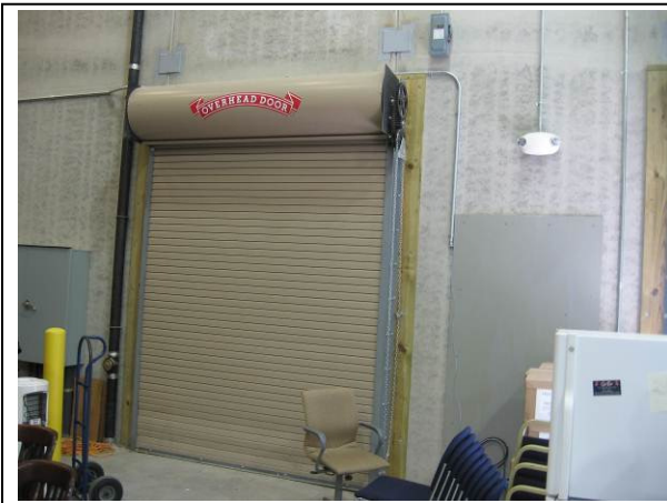
Photo 3: 02-22-13. Dauphin County Recycling Center. eWaste Recovery Program.
