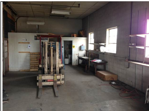
Photo 3: 02-15-13. Proposed Ewaste Building Building interior.
