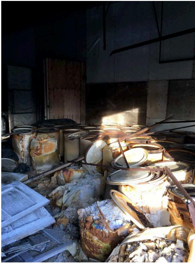
Interior of Pool Doctor business showing drums, deteriorating building conditions, collapsed roof, and unidentified waste.
