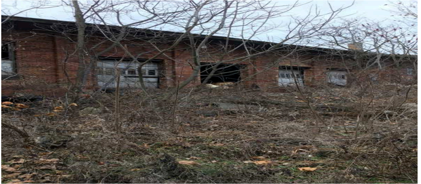
Pool Doctor building showing unrestricted access and drums of Solids in garage doorway
