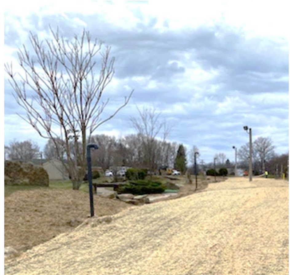
North LFG Collection Trench
