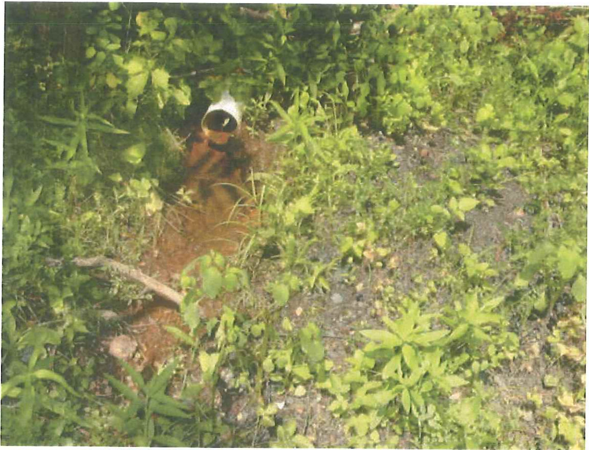
Picture #11 - Outfall from underdrain of landfill.
