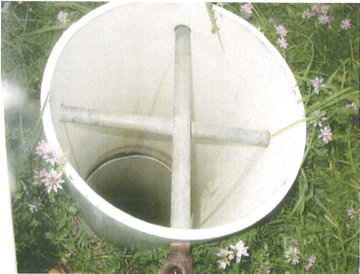
Picture #14 - Landfill cleanout.
