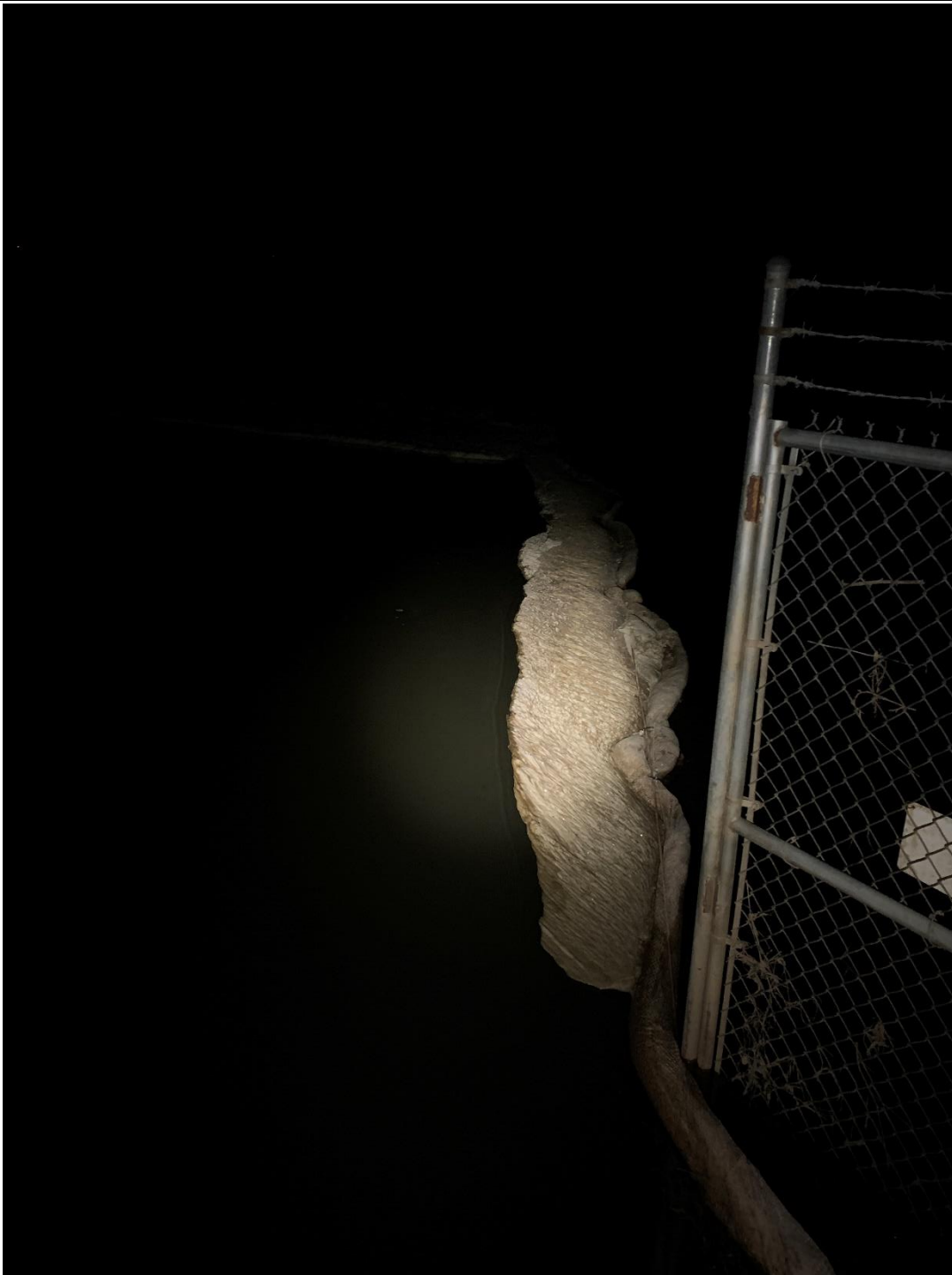
Photo #2 – Oil Boom Across the Mouth of the Channel
