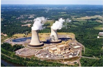
Limerick Generating Station
