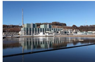
Peach Bottom Atomic Power Station
