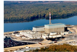
Quad Cities Generating Station
