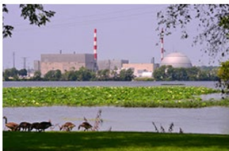
Dresden Generating Station
