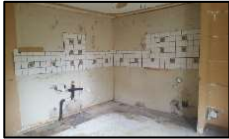
After RTP Cleanout
