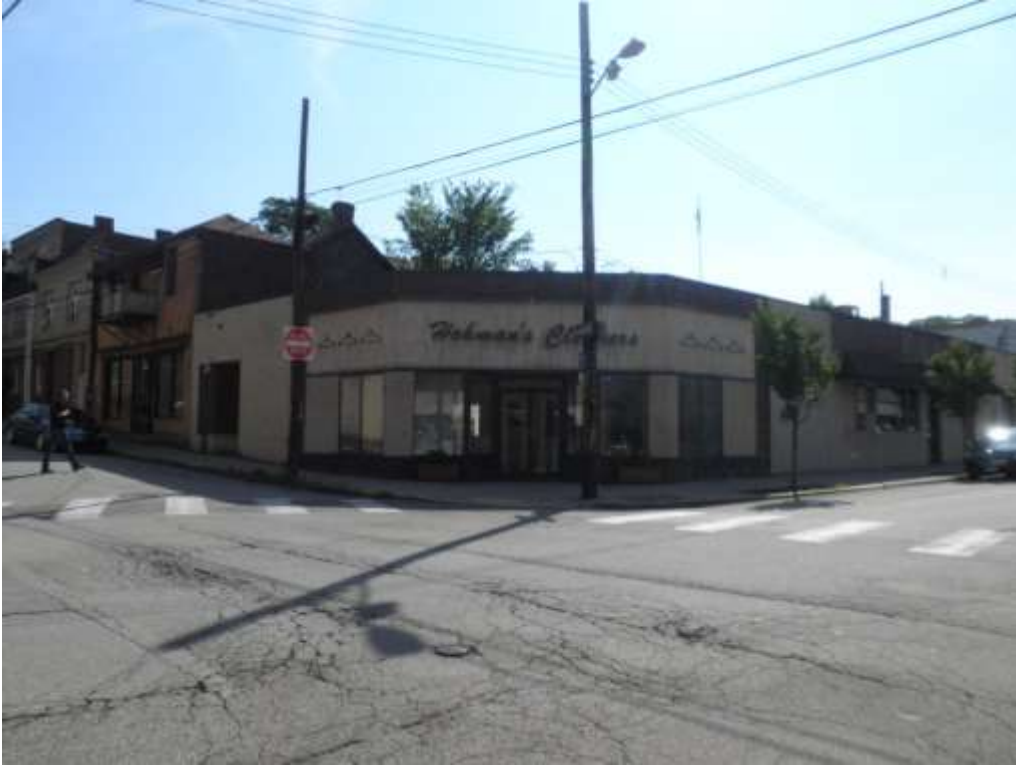
2105 Noble Street – Abandoned Dry Cleaners in Swissvale
