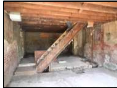
After Interior Demo
