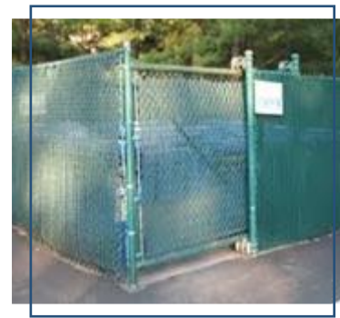
Small Site Adjacent to Municipal Building
