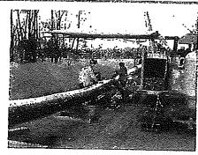
The welding crew begins the process of joining the steel pipe into long continuous segments. Welds are then radiographically inspected (X-rayed) to assure pipe joints have been welded in accordance with project specifications.
