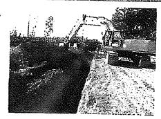
The trench is then **backfilled**. When soil conditions are not suitable to be directly placed on the pipe, specialized equipment designed to pad the pipe and protect it from sharp rocks and abrasion is utilized.
