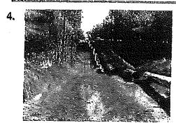
After the pipe is delivered to the right-of-way, the contractor "strings" segments of steel pipe by laying the pipe joints on wooden skids adjacent to the trench.
