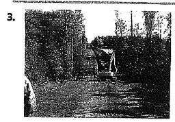
Next, the mechanical excavation of a trench, dug to a specified depth for pipe placement, is done by the **trenching** crew. Occasionally, rock drilling and blasting is required to break rock in a controlled manner.
