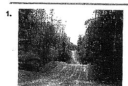
In order to make the right-of-way into a suitable work area, a **clearing and grading** crew prepares the pipeline corridor so the construction equipment can operate safely.
