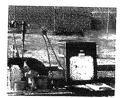
The newly constructed pipeline must be subjected to **pressure testing** before it can be placed into service. The purpose of a pressure test is to assure that no defects exist within the pipeline that might threaten its structural integrity. After the test, the pipeline is dried, cleaned and connected to the existing pipeline system.
