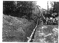
The pipe joints are cleaned and coated and the ditch bottom is cleared of rocks and debris or padded with soft dirt and the pipe is **lowered-in** to the ditch by sideboom tractors using belts or cradles in a carefully coordinated action. The ends of the pipe segments are then welded together to form one continuous pipeline.
