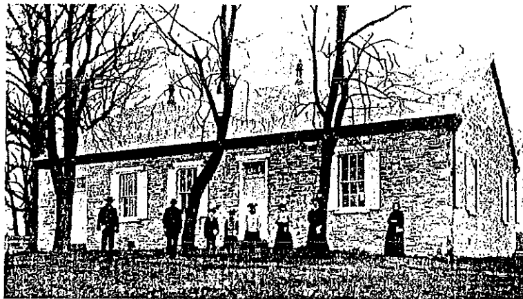
The River Corner Mennonite meetinghouse in southwestern Lancaster County was built in 1883. In Mennonites of Lancaster Conference (1931), historian Martin G. Weaver commented, "This meetinghouse is one of the most beautiful buildings of Colonial architectural design in the lower end of the county, and should be preserved for a long time." LMHS.
