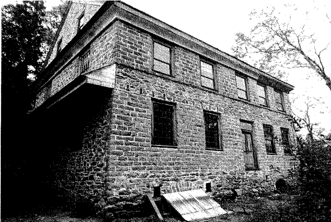
Photo 5: Southern elevation of Main Dwelling House, circa 1759
