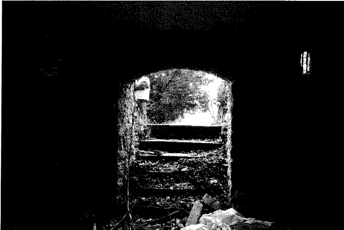
Photo 9: View from Main Dwelling House basement to exterior entrance looking south
