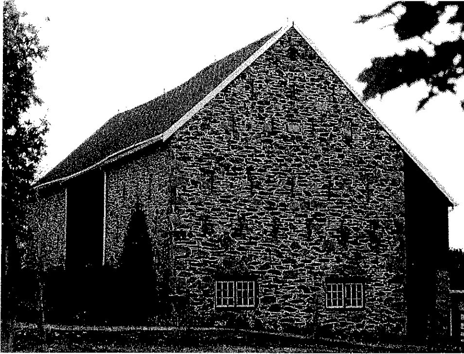
Photo 3: Shenk Barn (c. 1786), an excellent example of a well-preserved masonry Pennsylvania German Bank Barn (Herr 1992)
