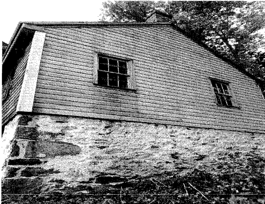
Photo 10: Eastern elevation of the 19 th -century Summer Kitchen
