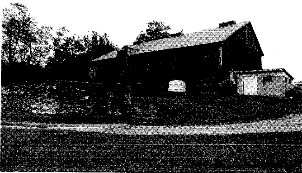
Photo 22: South and east elevation of Bank Barn; note intact Barnyard Wall in left foreground and mid-20 th -century Milk House to far right
