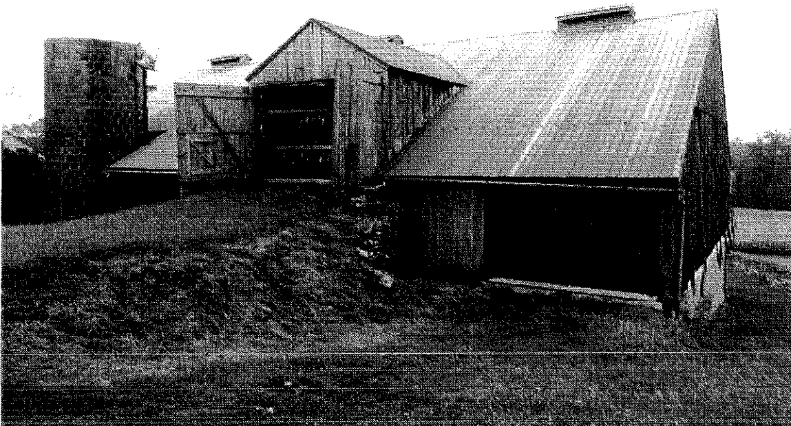
Photo 24: North and west elevation of Bank Barn, note active storage/curing of leaf tobacco
