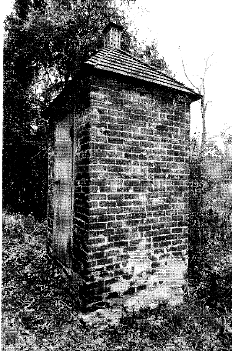
Photo 16: South and west elevation of Smoke House
