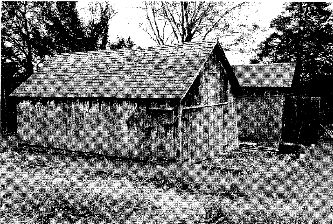
Photo 18: North and west elevation of 19 th -century Stables with Implement Shed in the background
