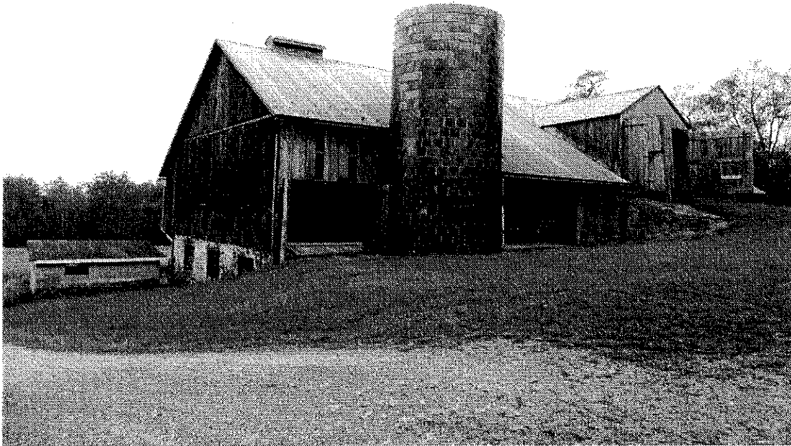
Photo 23: East and north elevation of Bank Barn, with adjacent early 20 th -century silo at center
