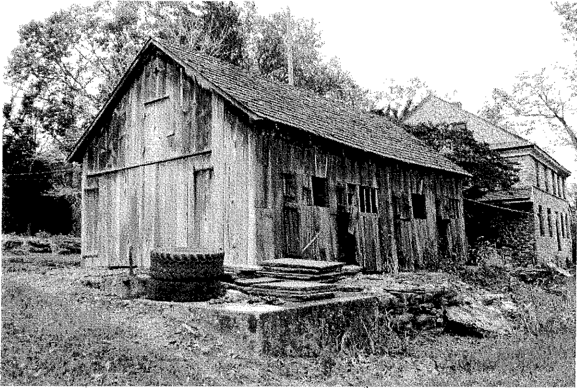
Photo 17: West and south elevation of 19 th -century Stables
