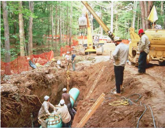
A side boom working on a cushion of soil in a narrowed ROW, L. Sauer
