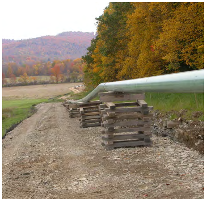
Construction of a natural gas gathering line pipeline, T. Carluccio
