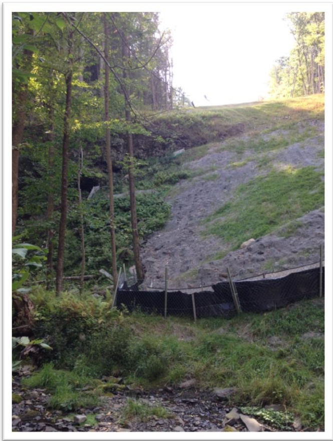
Sparse herbaceous growth, soil compaction, evidence of runoff and gullies, and sediment escaping the silt fences and traveling into adjacent Cummins Creek, an Exceptional Value Stream in Pike County, PA.
