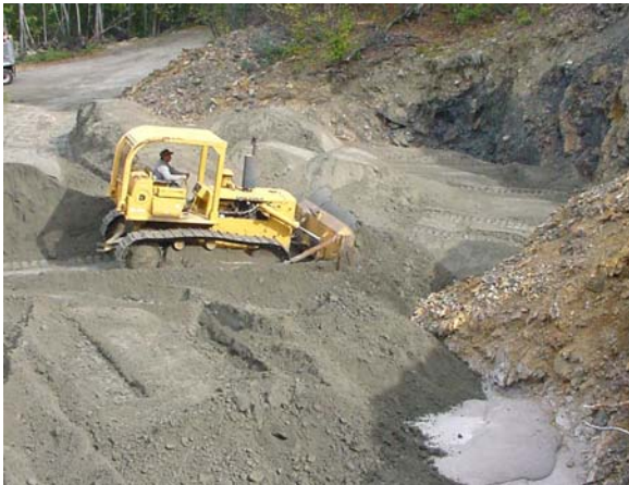
6.14(c). Ash bulk fill placed.
