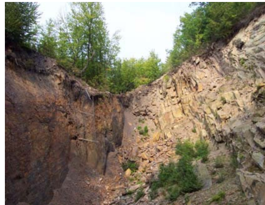
Figure 6.10(b). Expanding subsidence, notice the hanging chainlink fence on the left. Wall at the far end represents a stable pillar.
