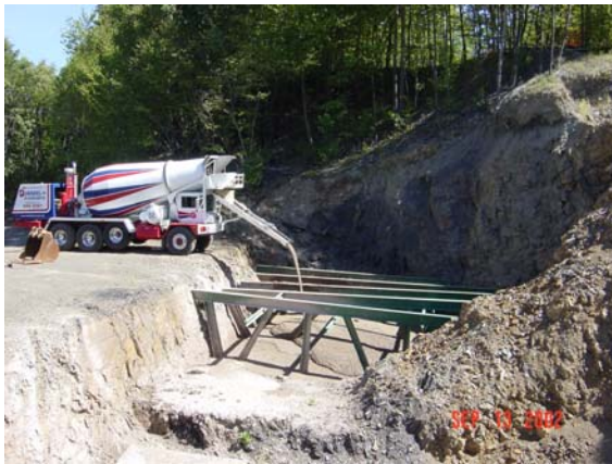
6.13(c). Grout mixture placement, Pit A east.
