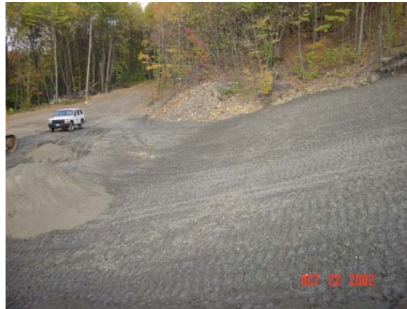
6.14(d). Prepared for topsoil. Pit A complete.
