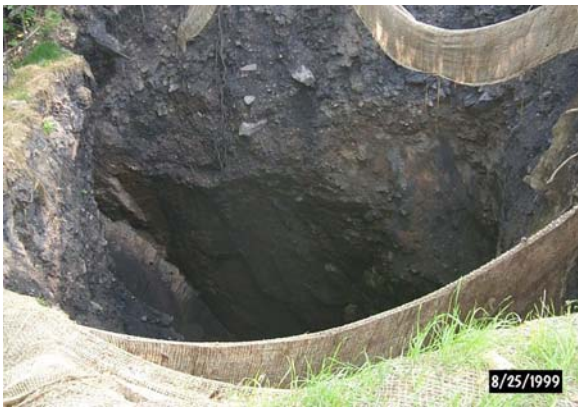
Figure 6.11(c). Severe collapse and loss of fill.
