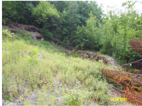
Figure 6.11(b). Sagging of filled area
