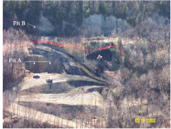
6.12(d). Demonstration Area, 2002. An orange safety fence surrounds the construction area.
