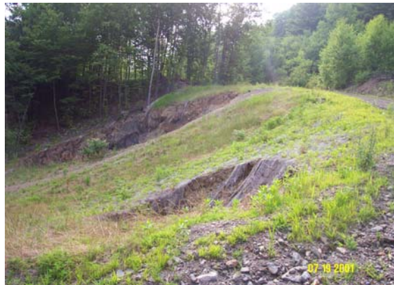
Figure 6.11(d). Subsidence. Site of Demonstration Pit A.
