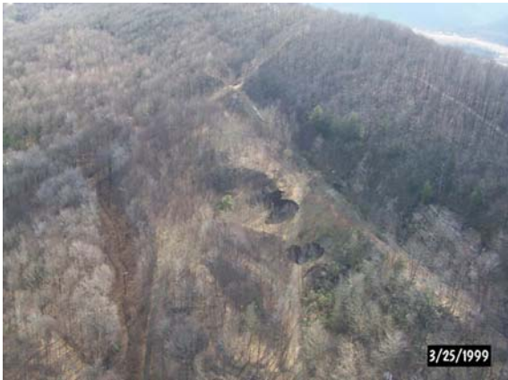
Figure 6.11(a). Emergency cropfalls.
