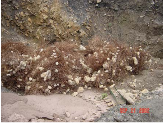
Figure 6.14(a). Scrap rebar in replaces trusses, Pit A west.
