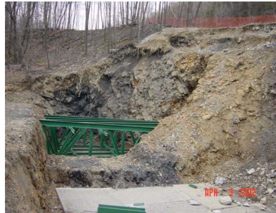
6.13(b). Steel trusses installed in Pit A east.
