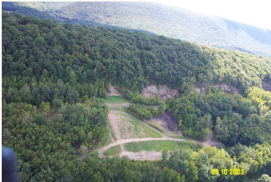
Figure 6.15. Completed Sharp Mountain demonstration project.
