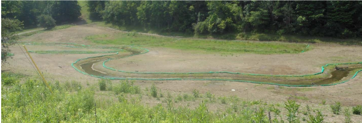
Figure VII-11. Photograph of the recently completed E20 gate cut on Crafts Creek. Banks had been re-shaped, but vegetation had not yet been planted. (Photo courtesy of A. Iannacchione).
