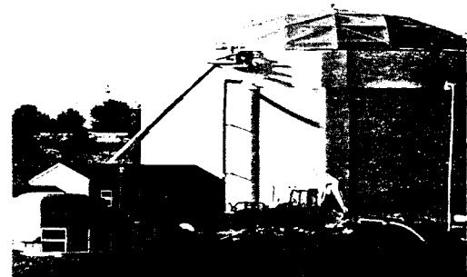
Work was progressing on installing a leachate pipe into the top of this one million gallon leachate storage tank. Pump stations and valve vault buildings are shown on the left which are used to control leachate being pumped to various tanks, truck couplings, and other pump stations throughout the GLRA landfill facilities. The leachate stored in this tank is pumped to the Lebanon City Waste Water Treatment Plant via the North Lebanon Township sewer system.
