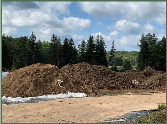
Excavation area with Black Moshannon Lake in the background September 2022
