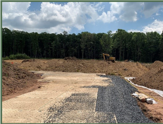
Excavation activities August 2022
