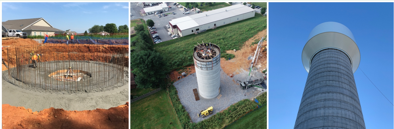
500,000 Gallon Water Tower (Left to Right) Foundation, Mid Construction, Completion
