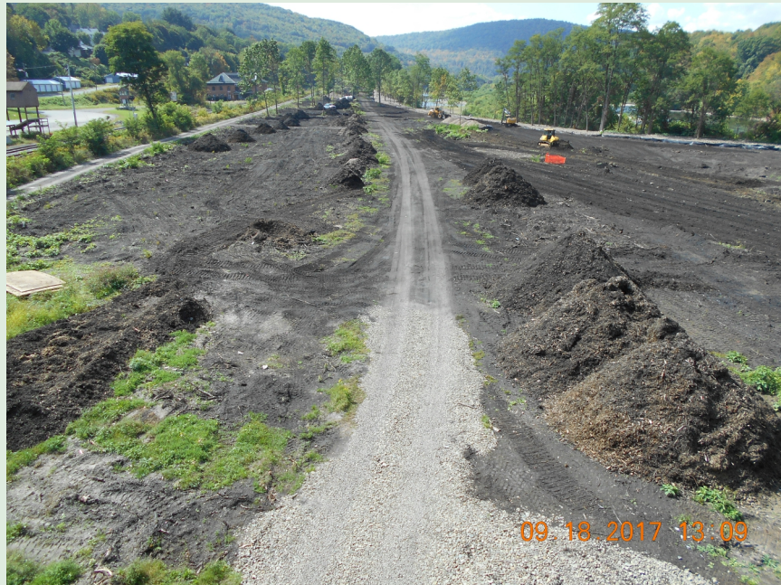
September 2017 After Clearing and Grubbing
