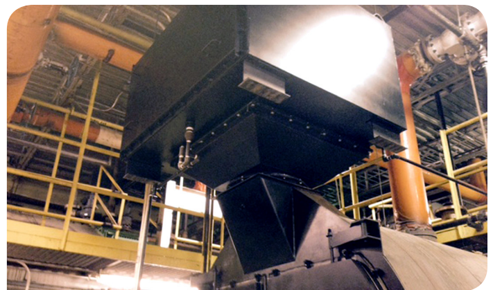
Left: The burner is controlled electronically and manages the flame to ensure maximum fuel output of the boiler.
